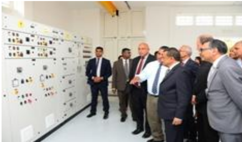
Visit to Pumping station Pailles
