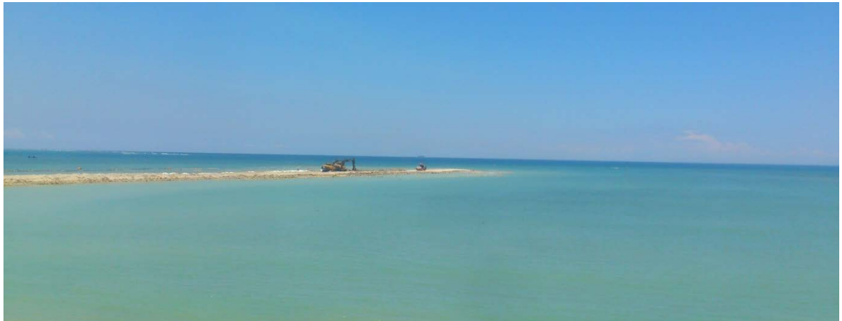
Exhibit 4-19 Ongoing reclamation works – 2
