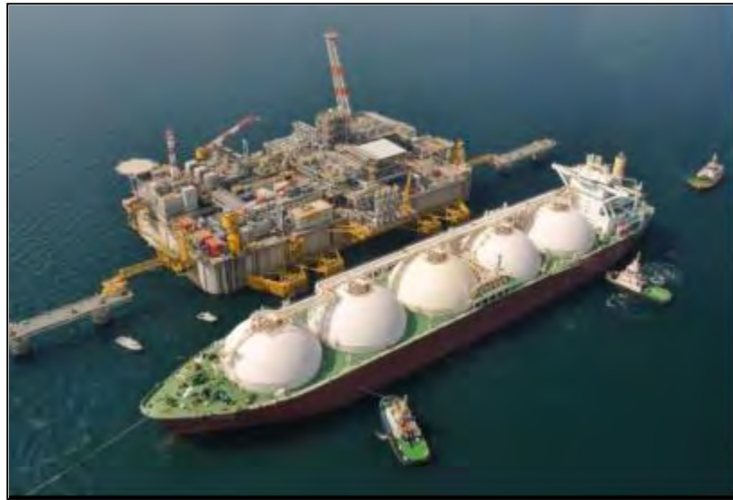
Exhibit 3-35: Gravity Based Structure – Concrete
