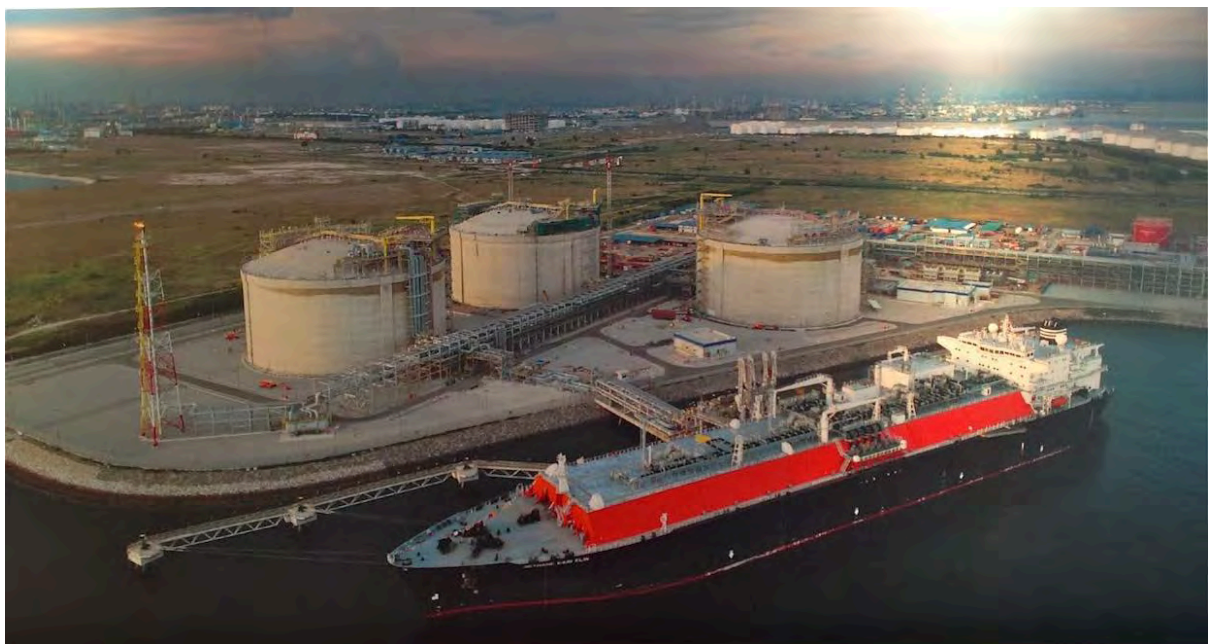
Exhibit 3-3 Shore based LNG terminal (Singapore LNG)
