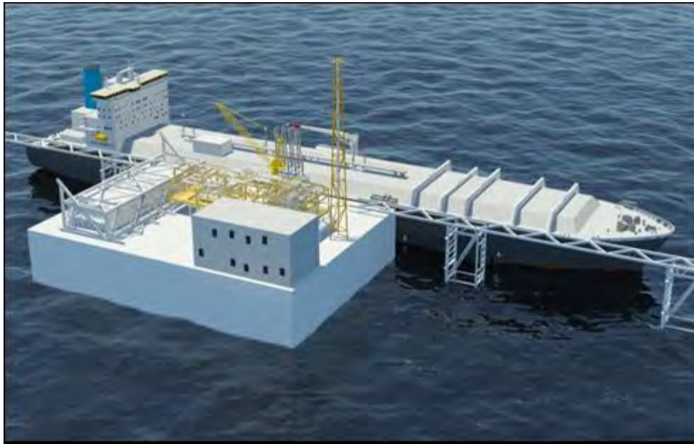
Exhibit 3-36: Gravity Based Structure – Steel
