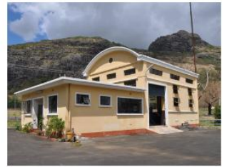
LA FERME HYDRO POWER STATION
