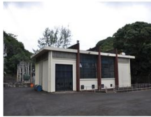
CASCADE CECILE HYDRO POWER STATION
