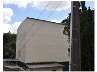
MAGENTA HYDRO POWER STATION
