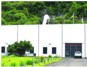
CHAMPAGNE HYDRO POWER STATION
