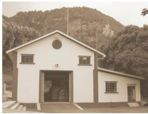
LE VAL HYDRO POWER STATION
