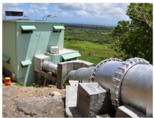
LA NICOLIERE FC HYDRO POWER STATION
