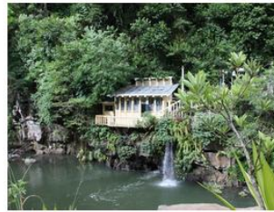
A.I. ATCHIA POWER STATION
