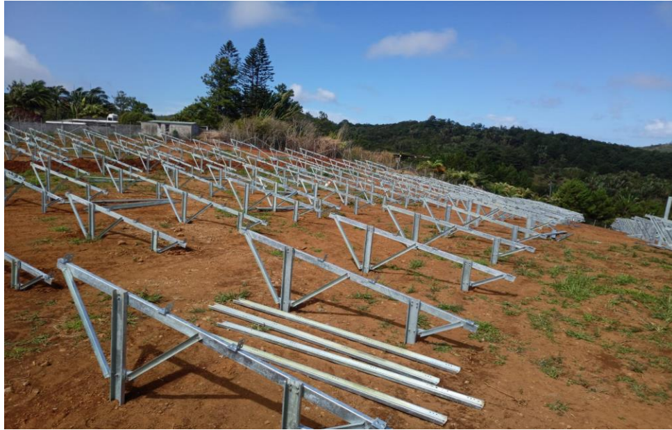
Figure 2: Construction of the Solar PV Farm
